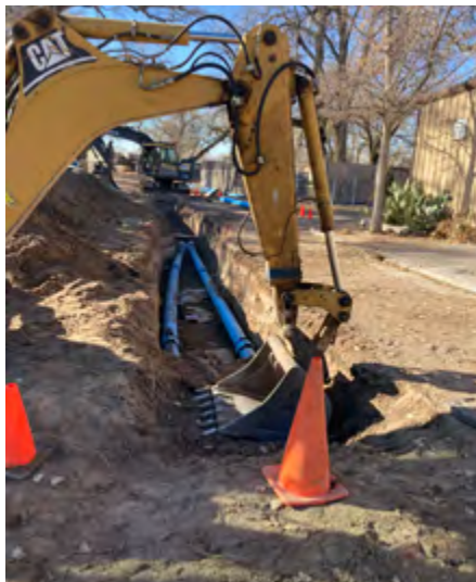
City of Albuquerque BioPark Utility Expansion, Albuquerque, NM
