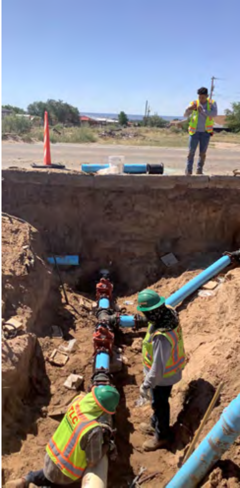
Ohkay Owingeh Water Conveyance Project, Pueblo of Ohkay Owingeh, NM
